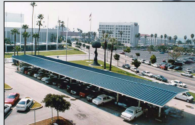
30 kW Parking Shade Structure
